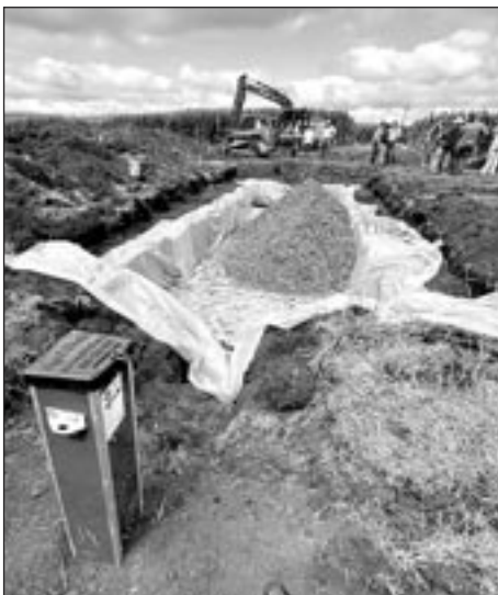
Water sampling stations are located at either end of the denitrifying bioreactor.
